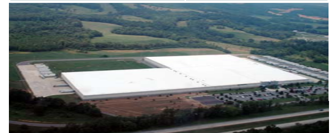
Ferguson Distribution Center
