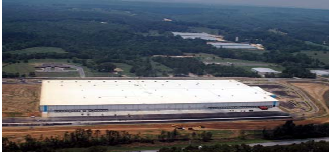
The Children's Place Distribution Center
